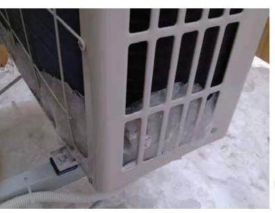
Without the right technology, condensate freezes to the bottom of the unit and reduces its efficiency and heating output.
